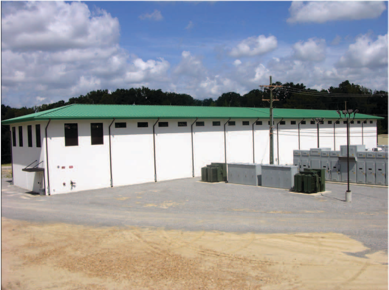
ERDC DSRC new 10,000 sq ft computer room
